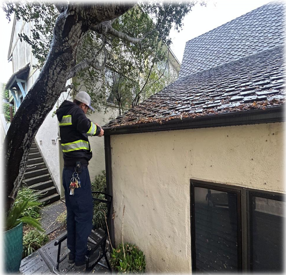
City Hall Gutter Repair
