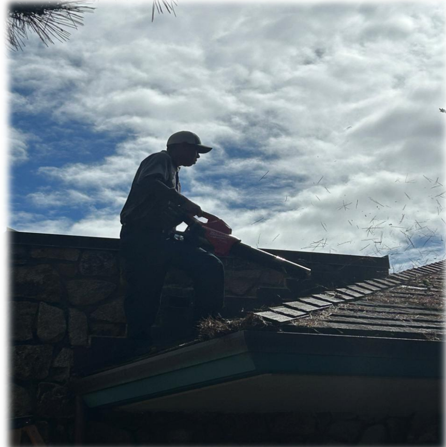
Children's Library Roof and Drainage Cleaning
