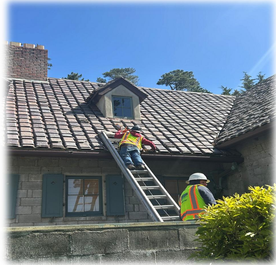
Flanders Mansion Leaky Roof Repair
